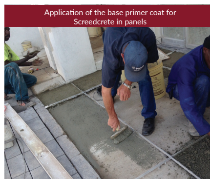
Mauritius hotel external walkways.
